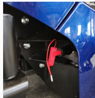
Fig. 96: Battery dicon. switch, inactive
